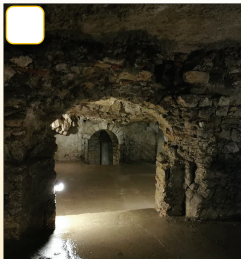
People discovered the underground passages and turned them into cellars.
